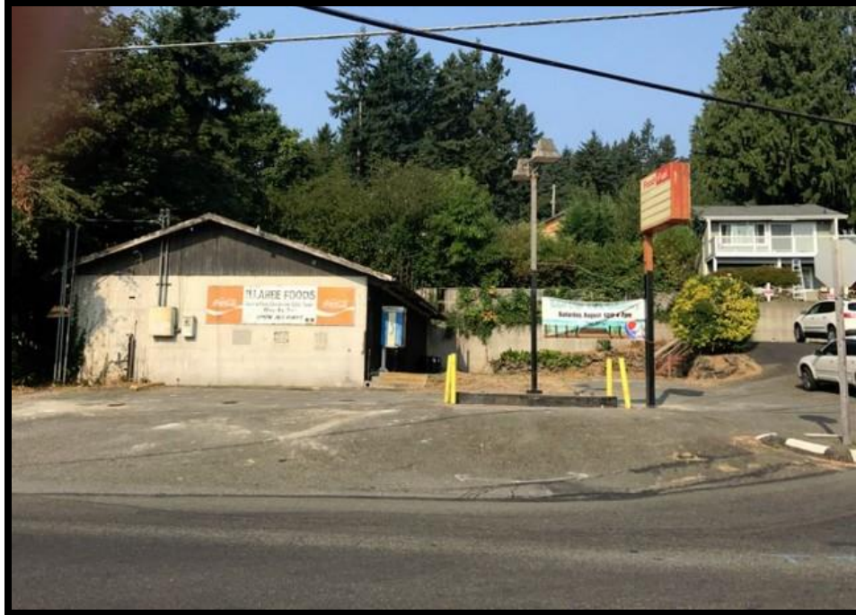
1) View of subject, looking west.
