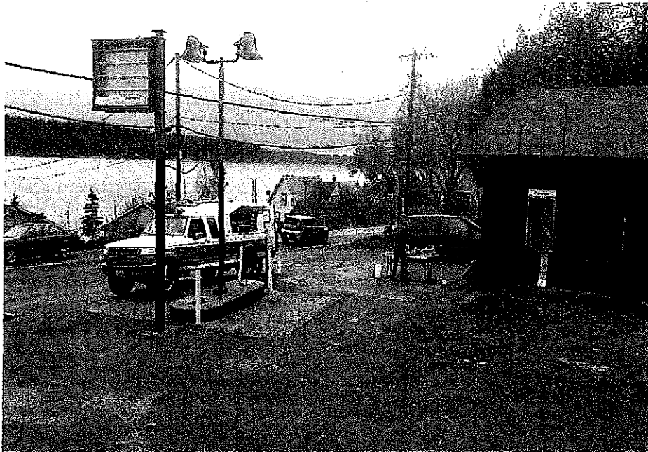
Looking south at the former fueling/dispenser location. Sampling table set up on UST pit area.
