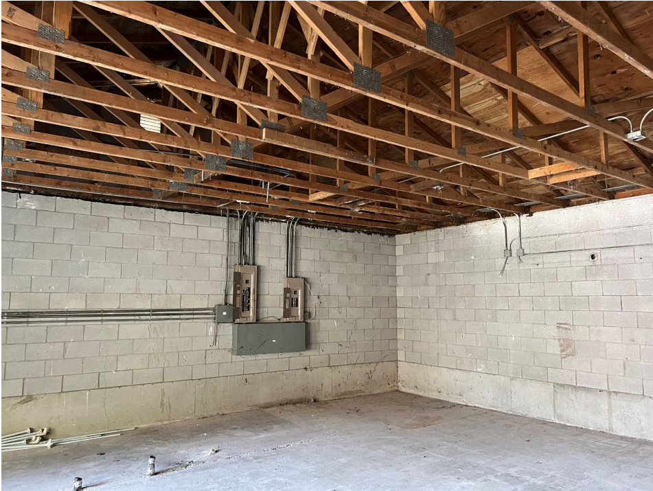
Interior southeast corner, existing elec. panel and sink drains:
