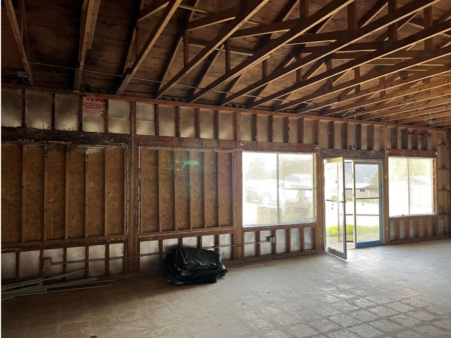
Interior north wall:
